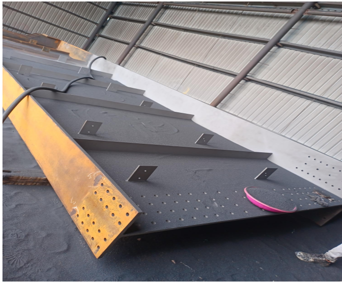
Covered Surface preparation area
