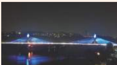
Durgam cheruvu cable stayed bridge , Hyderabad, clicked by Molina d/o Nagesh, Dy. Manager (BMS Dept.) Corp. Office
