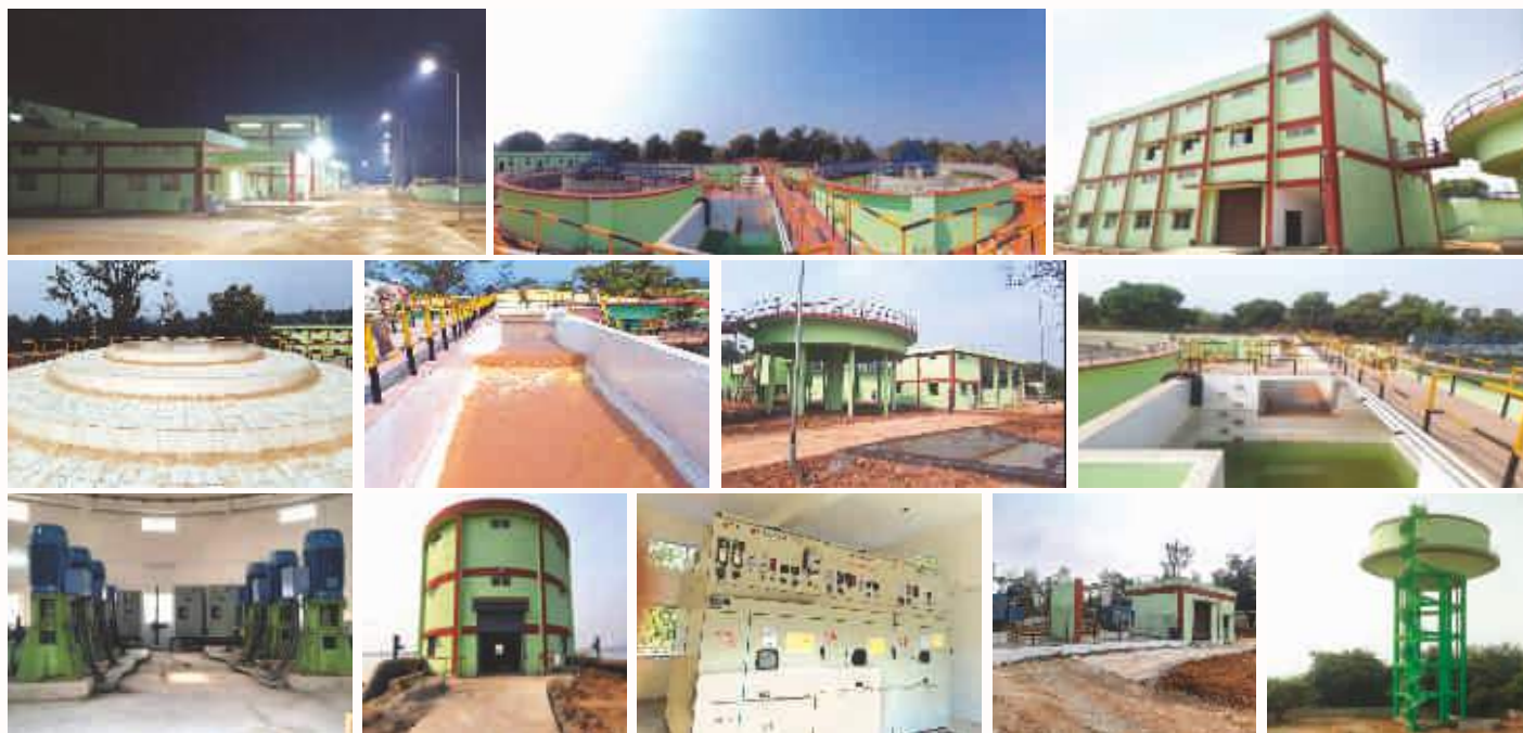
Intake Well Cum Pump House
